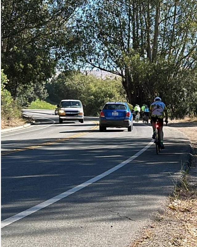
Class II bike lanes (Existing condition on S Bay Blvd)
