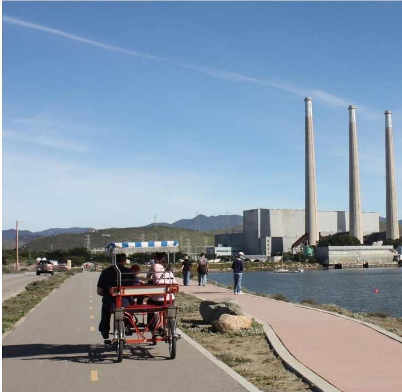
Class I with horizontal separation from roadway
