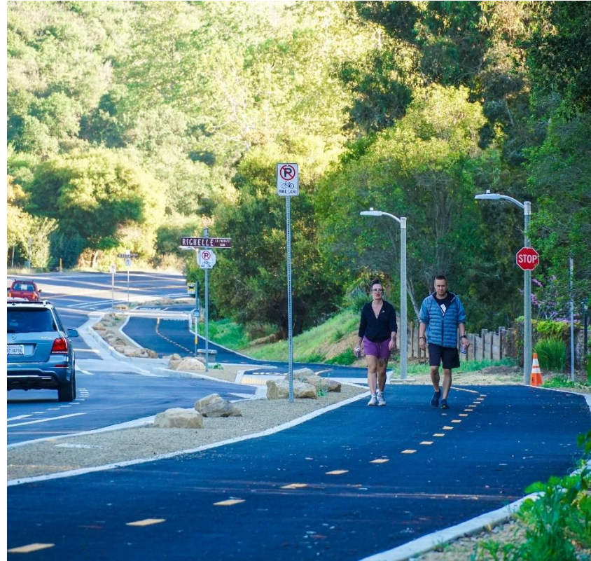
Class I with horizontal separation from roadway
